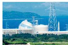
Genkai Nuclear Power Station (Saga Prefecture)
