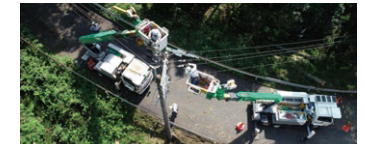
Restoration work underway
