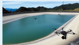
Drone footage of a dam wall
