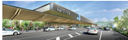
Kumamoto Airport privatized operations business (New terminal building to be in service in March 2023)
