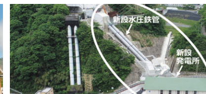
Replacement work at the Tsukabaru Hydroelectric Power Station
