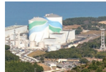
Sendai Nuclear Power Station (Kagoshima Prefecture)
