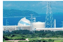
Genkai Nuclear Power Station (Saga Prefecture)
