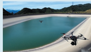
Drone footage of a dam wall
