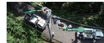
Restoration work underway
