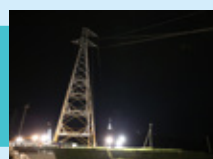
Restoration work following Kumamoto Earthquake
