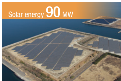
Solar energy 90 MW Mega Solar Omura Power Station Units 1-4 Location: Nagasaki Prefecture Capacity: 17.48 MW (panel capacity: 20.35 MW) Start of operations: March 2013
