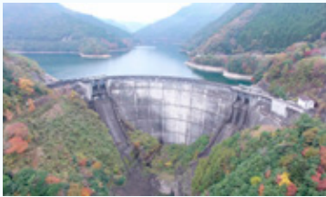
Japan's first arch-type dam [Kamishiiba Power Station]
