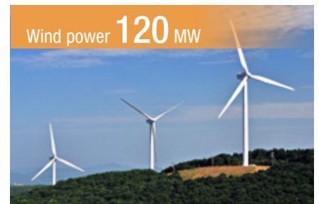
Wind power 120 MW Nagashima Wind Power Station Location: Kagoshima Prefecture Capacity: 50.4 MW Start of operations: October 2008
