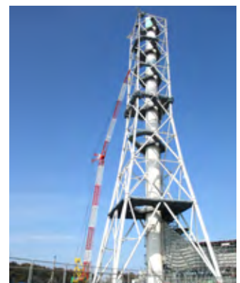
Shin Oita Unit 3 (Axis 4) construction site
