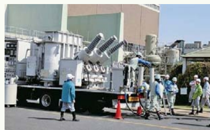
Drill to restore an external power source
