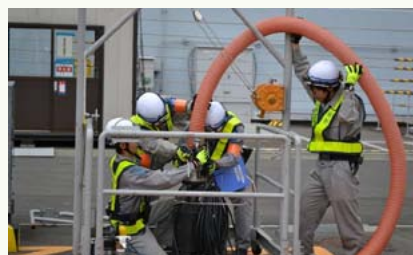
Drill to supply coolant water with a temporary pump
