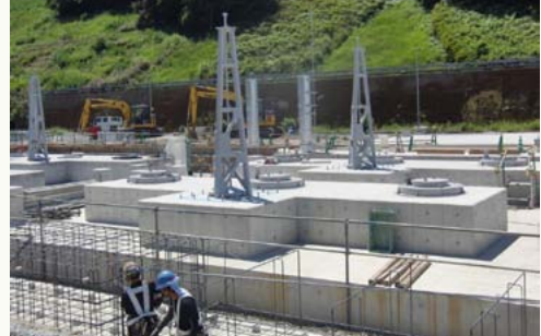
Construction of additional fuel tanks to emergency diesel generators
