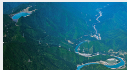
Omarugawa Power Station (Miyazaki)
