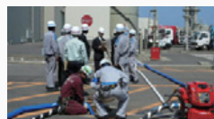
Practice drill on supplying coolant water with temporary pumps
