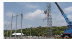
Practice drill on temporary restoration of pylons, etc.
