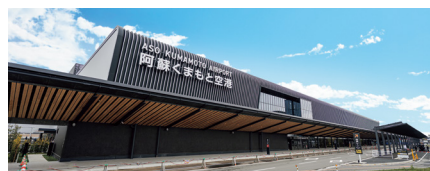
Kumamoto Airport privatized operations business (new passenger terminal building) (Opened for public use in March 2023)
