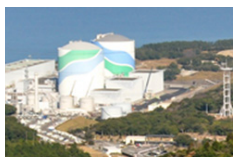
Sendai Nuclear Power Plant (Kagoshima Prefecture)
