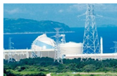
Genkai Nuclear Power Plant (Saga Prefecture)
