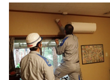
Indoor wiring inspection (Kumage Distribution Office)
