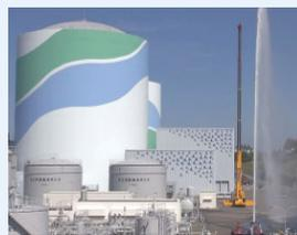
Discharge test using a water cannon
