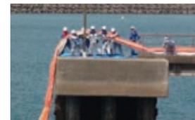
Drill involving the establishment of a silt fence (in-sea curtain)
