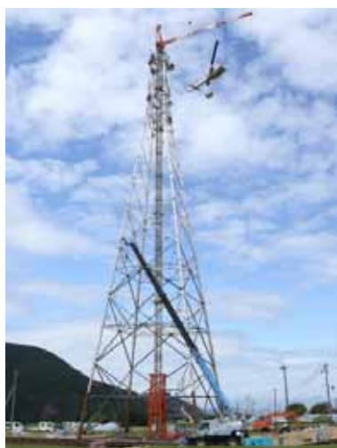
Wiring of temporary steel tower
