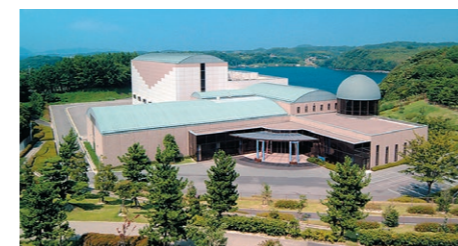
Exterior view of the Nuclear Power Training Center
