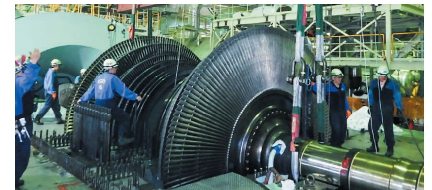
Overhaul inspection of turbine
