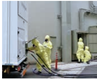
Connecting power cables from a high-voltage generator truck
