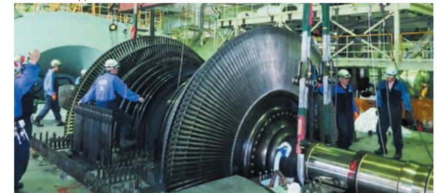
Overhaul inspection of turbine
