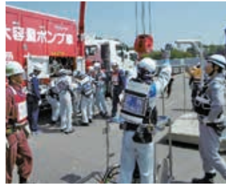
Connecting a high-capacity pump truck
