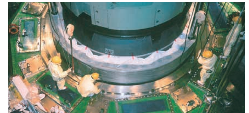
Removal of upper head of the reactor vessel
