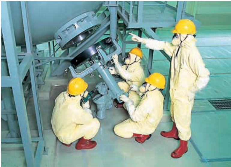
Steam generator water chamber mock-up (Training in opening, inspection and restoring the steam generator water chamber.)
