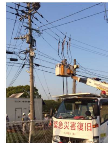
[配電線復旧作業]
